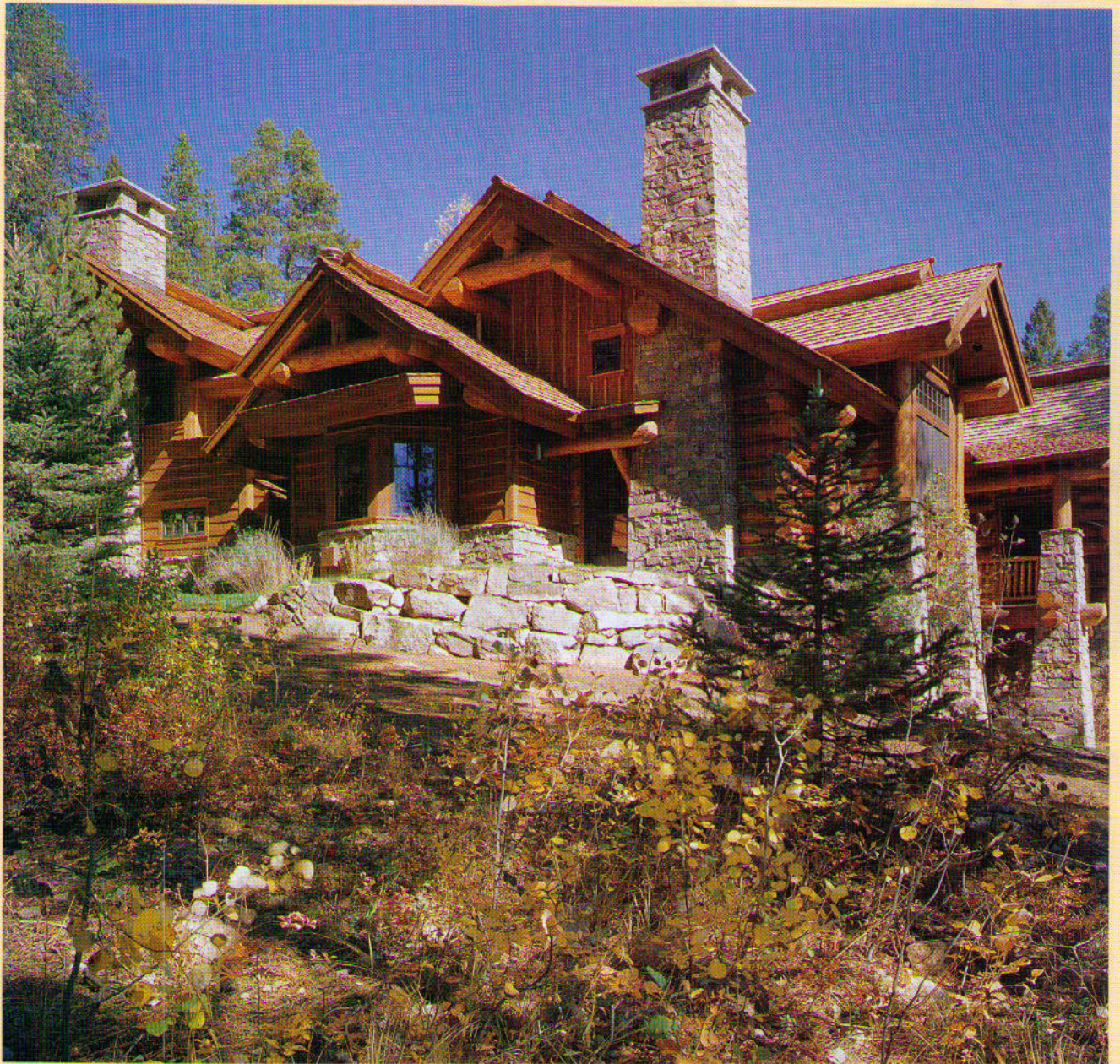
Multiple rooflines and stone piers supporting log columns help this home conform to the landscape. Its rambling look is intended to convey the impression that the home was originally a small cabin that has been added onto over the years.
