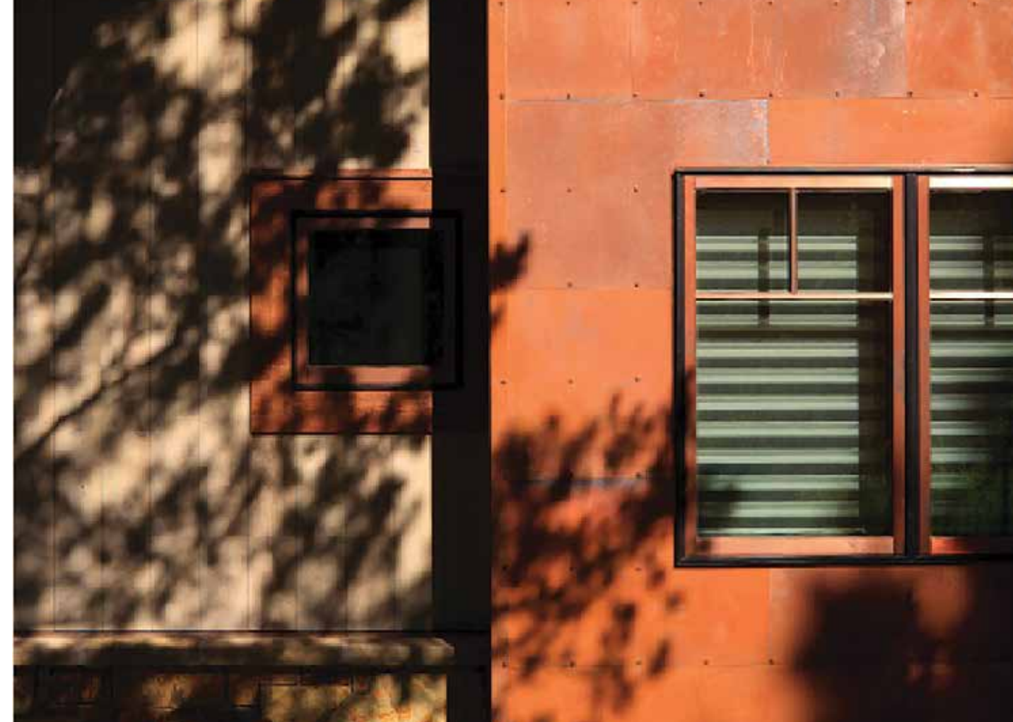
THIS PAGE Teton Heritage Builders is pleased with the performance of steel cladding, so much so, they clad their own office. PHOTO Courtesy of Teton Heritage Builders. OPPOSITE, UPPER Finishes change the character of steel cladding, as exemplified by this oxidized treatment by Teton Heritage Builders. PHOTO Courtesy of Teton Heritage Builders. OPPOSITE, LOWER A mix of wood slats and riveted oxidized steel reflect a daring design ethos. PHOTO Courtesy of Atelier One Ltd.
