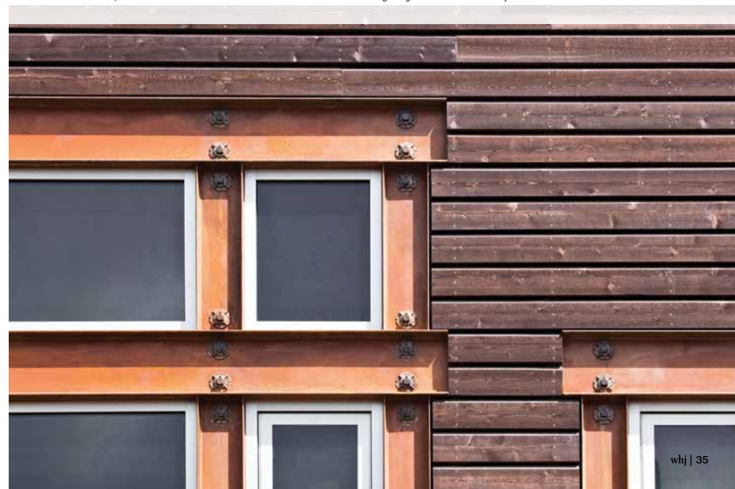
THIS PAGE Teton Heritage Builders is pleased with the performance of steel cladding, so much so, they clad their own office. PHOTO Courtesy of Teton Heritage Builders. OPPOSITE, UPPER Finishes change the character of steel cladding, as exemplified by this oxidized treatment by Teton Heritage Builders. PHOTO Courtesy of Teton Heritage Builders. OPPOSITE, LOWER A mix of wood slats and riveted oxidized steel reflect a daring design ethos. PHOTO Courtesy of Atelier One Ltd.
